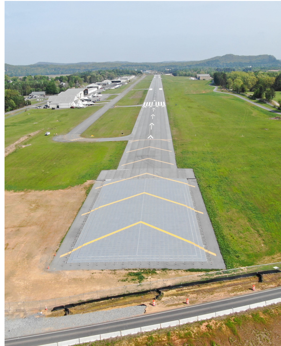
Cartersville 2 nd EMAS Project Thomaston - Upson County Airport
